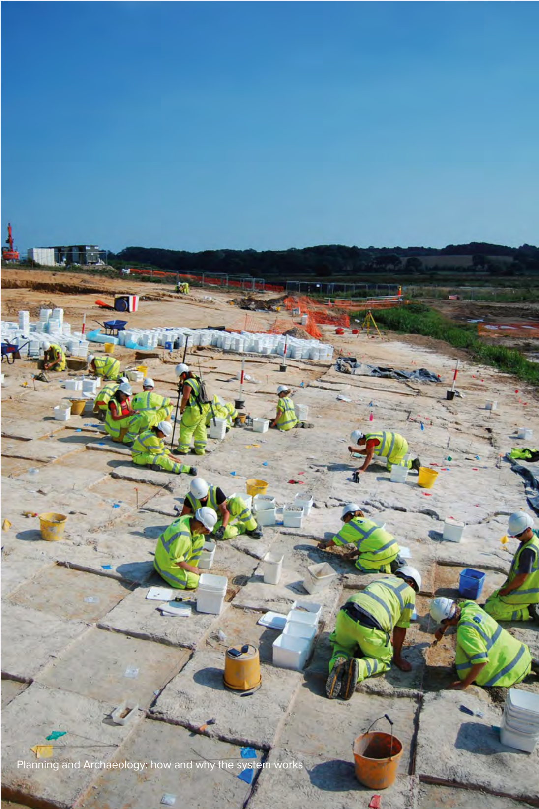
Excavations in progress on the Bexhill to Hastings Link Road. © Oxford Archaeology
